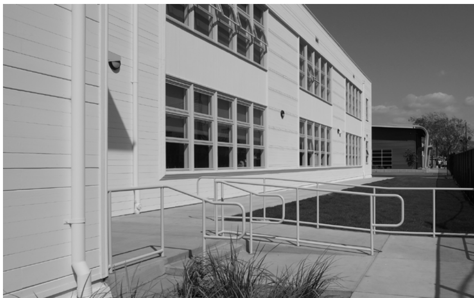
Figure 3: Detail of the rehabilitated building showing the unique siding pattern. September 2016.
